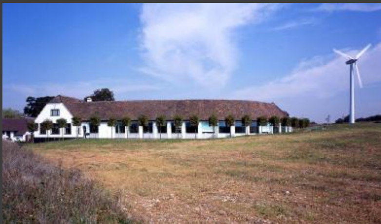
Credit: Studio E Architects
